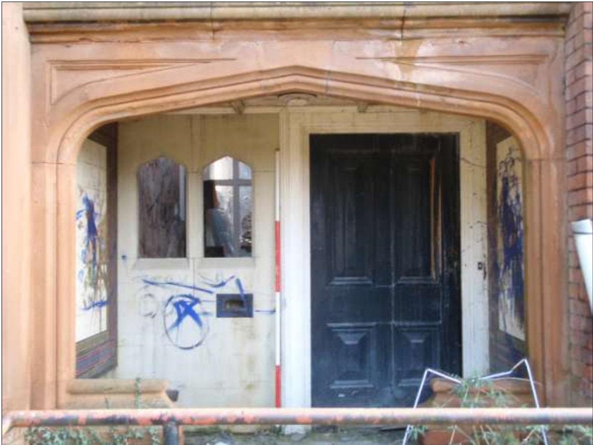
Figure 7. The main entrance is framed by a four-centred Tudor arch with carved spandrels in red sandstone leading to a framed fielded panelled door finished in black paint. To the left of the door an off-white stone fielded panel with two Tudor arched windows with later letter box. Two framed pictorial tiled inserts are to be seen on the porch walls left and right of the main door. Both have been vandalised by sprayed paint (2m scale).
