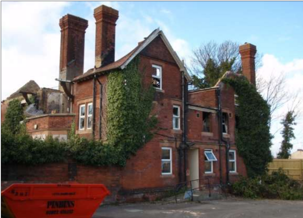
Figures 12, 13 Rear of property (facing west) show both gables, windows with red sandstone sills and lintels. South side of the house, (below) showing mullioned bay construction. Scale in 50cm sections.
