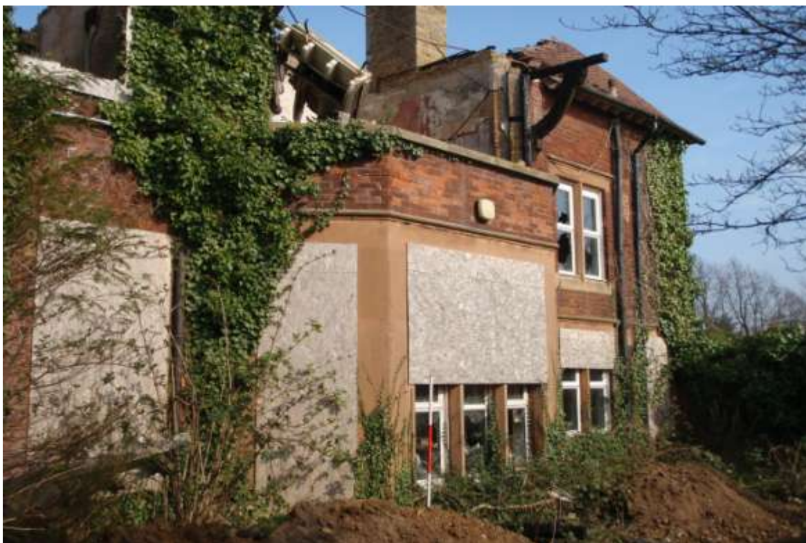
Figures 12, 13 Rear of property (facing west) show both gables, windows with red sandstone sills and lintels. South side of the house, (below) showing mullioned bay construction. Scale in 50cm sections.
