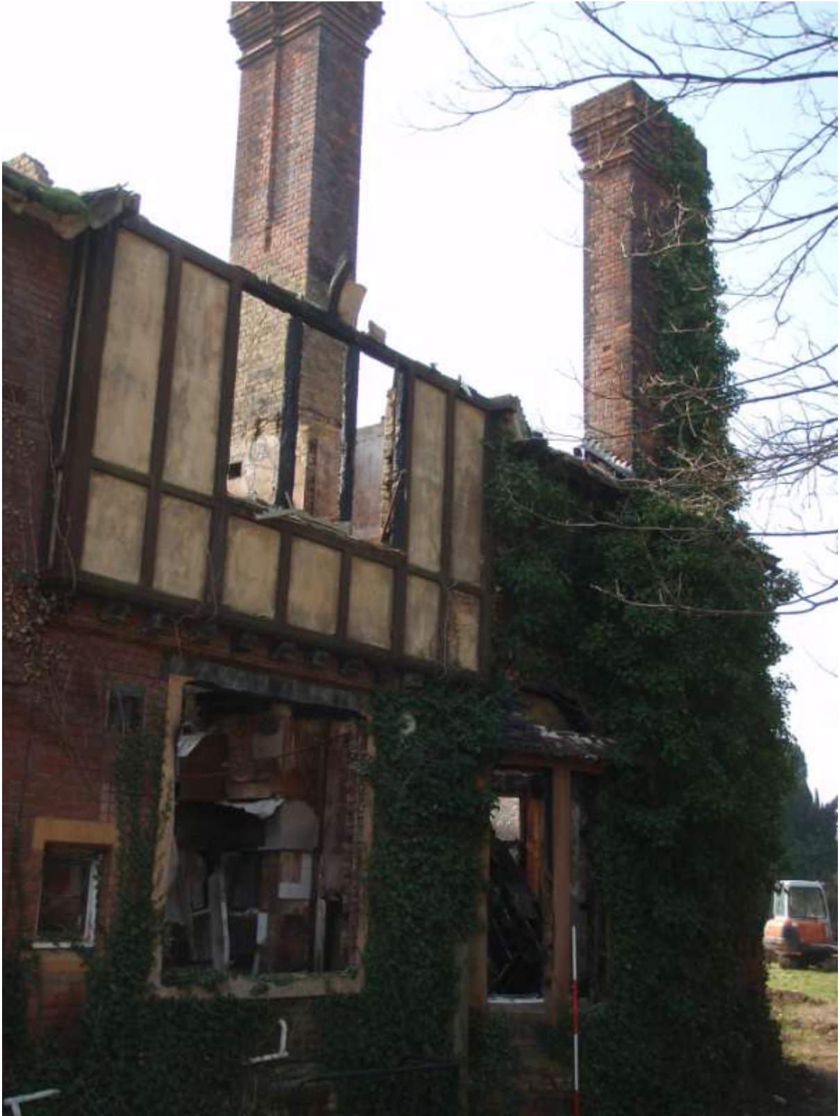
Figure 14. Showing north side of the house with timber-framed jettied upper storey in Elizabethan- style with three-light mullioned window. Infill panels are finished in off-white lime mortar. Below on the ground floor the windows are framed in red sandstone.
