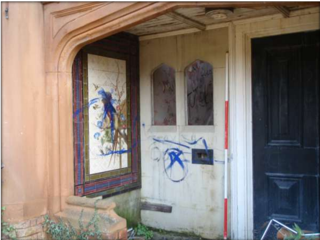
Figure 5. Front porch built of fine red sandstone in the Tudor style and located on the west front with two inset tile panels (2m scale).
